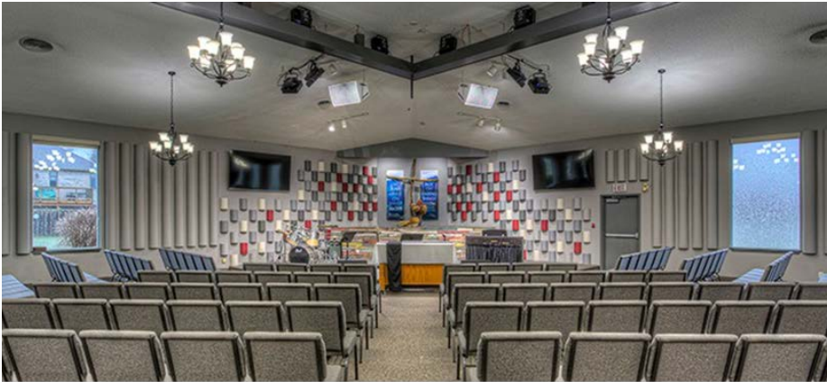
Figure 4 A creative implementation of diffusers at Tillsonburg Alliance Church in Ontario.
